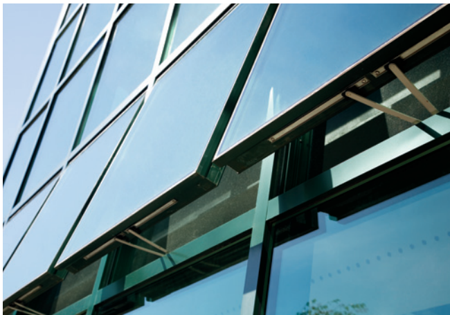
Massanutten WaterPark, Massanutten, Virginia, USA Architect: Dembling + Dembling Architects, P.C., Albany, New York, USA Glazing Contractor: Architectural Glass & Mirror, Clifton Park, New York, USA
