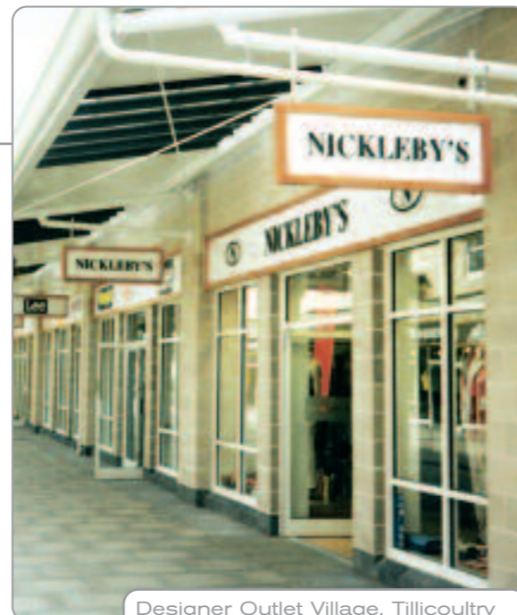
Designer Outlet Village, Tillicoultry Architect: Dalziel Design Partnership
