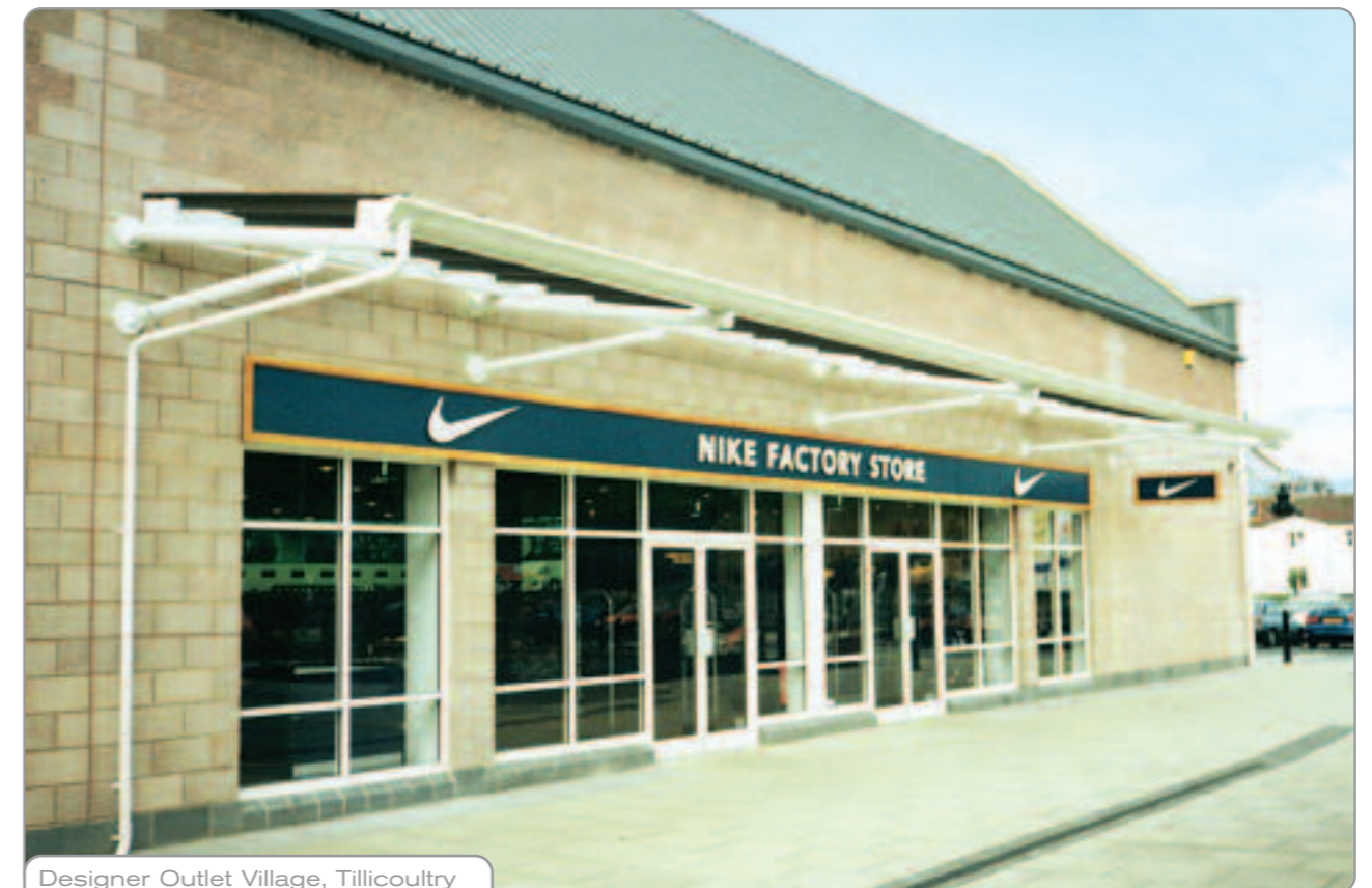
Designer Outlet Village, Tillicoultry Architect: Dalziel Design Partnership
