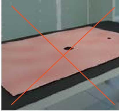
WRONG: NO SURFACE ACTIVATOR SILICONE
