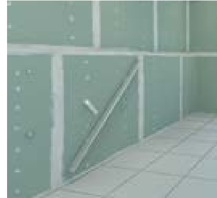
MEASUREMENT OF FLATNESS OF THE WALL
