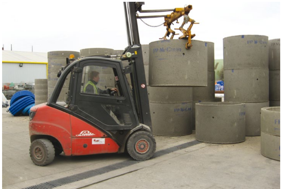
The heavy duty channel drainage system met the hydraulic demands of the site.
