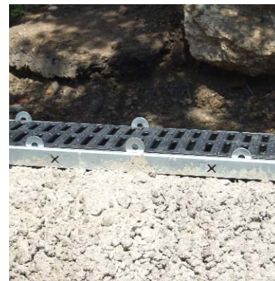
Fig.2 Washers are used to aid grating removal
