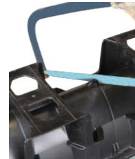
Cutting guide for 0.5m channel units
