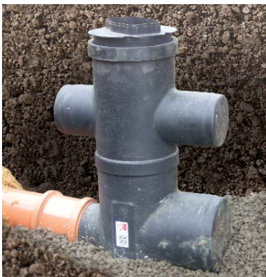
Fig.1 Sump unit connected to the outlet pipe
