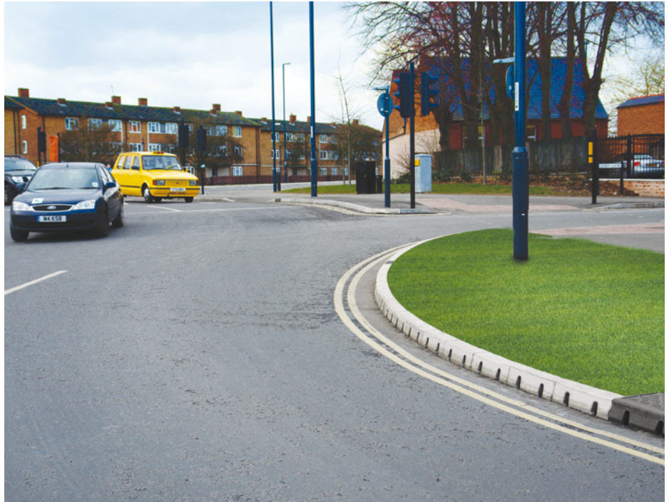
The combination of ACO KerbDrain radius and drop kerb creates a seamless and continuous kerblines across the entire project.
