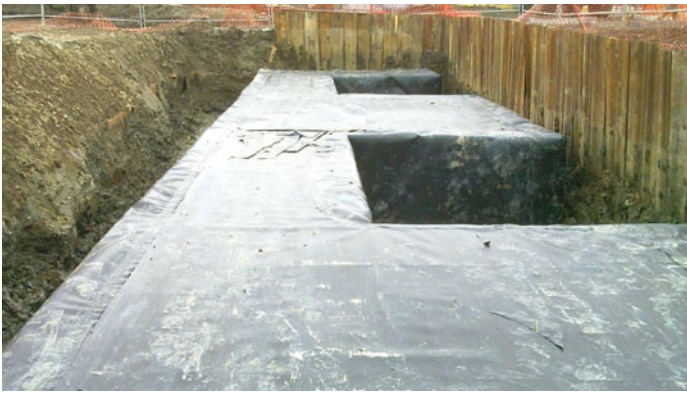
The recesses formed on the roadside edge of the installed ACO StormTank accommodate the parking bays and avoid any direct, vertical loading.
