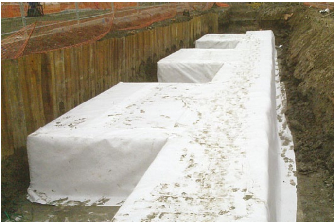
The polypropylene fleece that forms the outer layer of the ACO StormTank installation protects the integrity of the inner waterproof liner.
