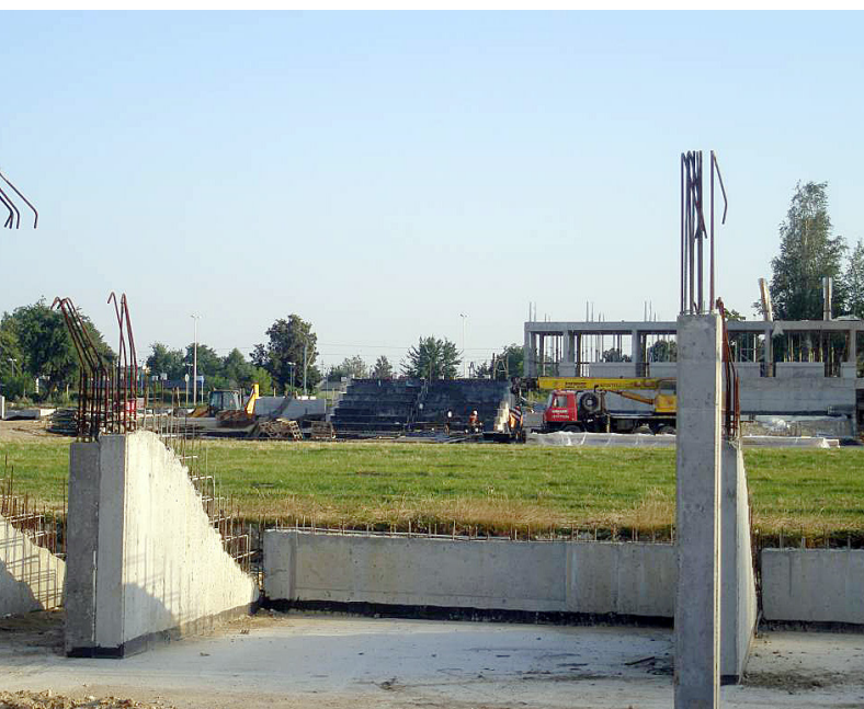
Current status of construction (August 2013)
