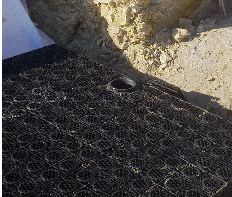
ACO Stormbrixx – assembly – as a tie-in to the access chamber system
