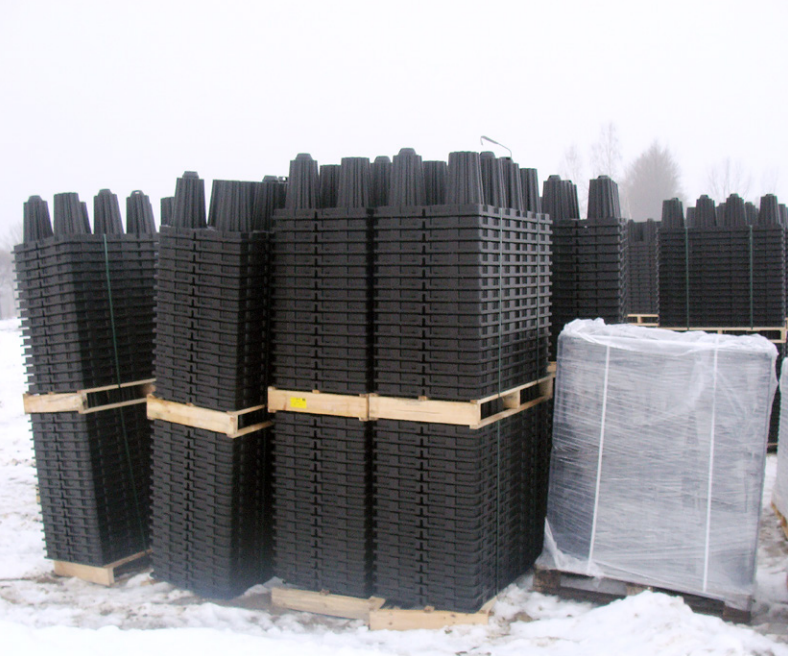
ACO Stormbrixx delivered to the construction site – first batch of goods.
