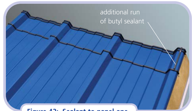
Figure 42: Sealant to panel one
