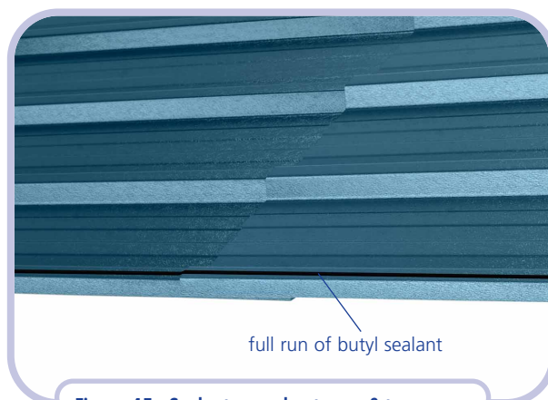
Figure 45: Sealant over sheets one & two
