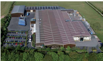
Warnell facility, Carlisle
